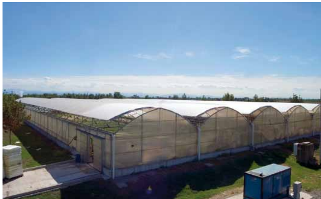
Serre alimentate a biogas
